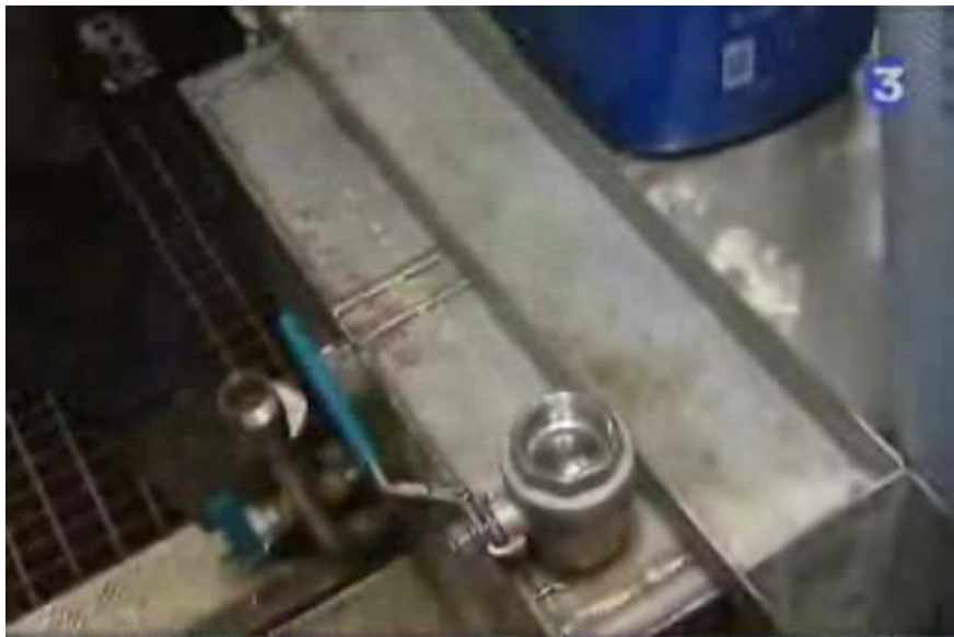
Water Feed GEET variant boat installation
